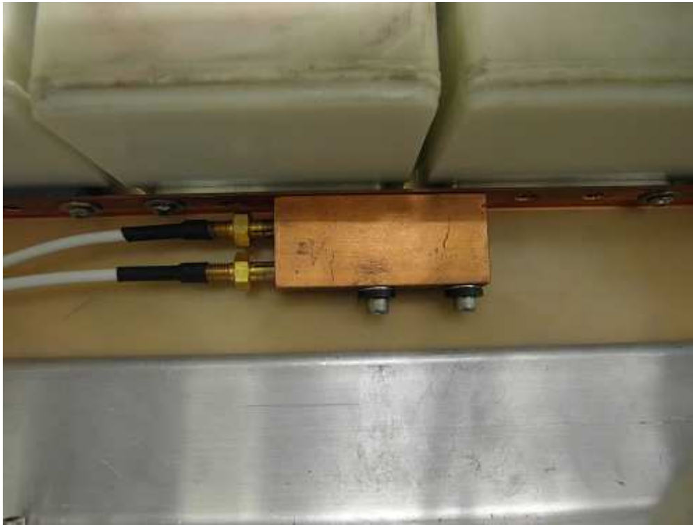
Figure 3.11 Capacitor bank interconnects.
